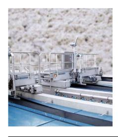
Automatic and turbulence-free removal of grit sediment and floating scum, which accumulate as a result of solids separation in chambers during grit and grease removal process in wastewater treatment; thereby preventing issues with downstream processes.
