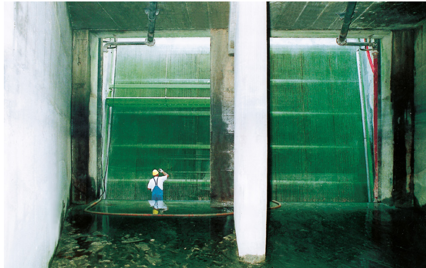
Passavant®/Geiger® COB Screens. View on the channel bottom
