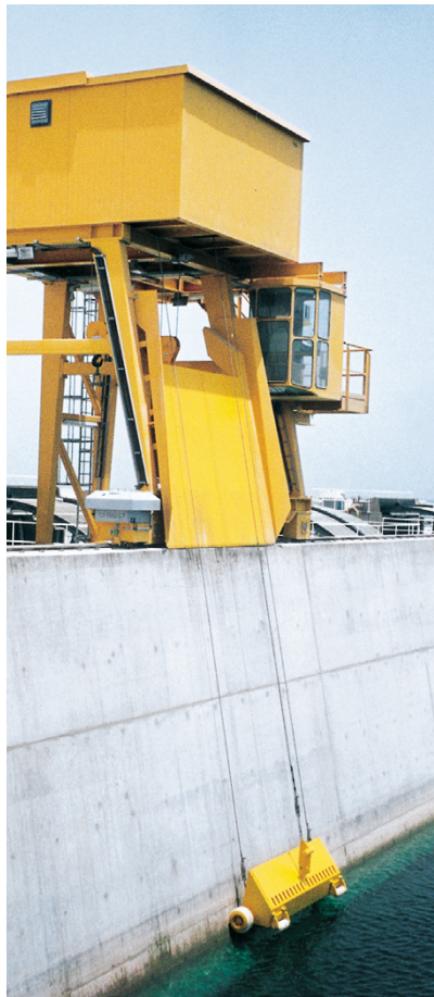
Picture on the left: Passavant®/Geiger® Traversing Cable-Operated Bar Screen in Action
