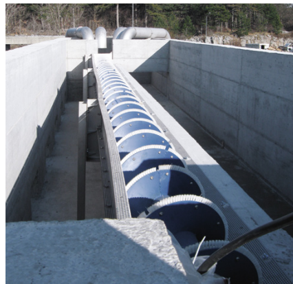
OVF 300 Stormwater Overflow-Screening of mixed effluent
