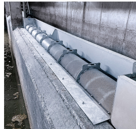
OVF-R 300 Stormwater Overflow-Screening
