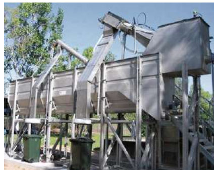
Municipal wastewater treatment plant
