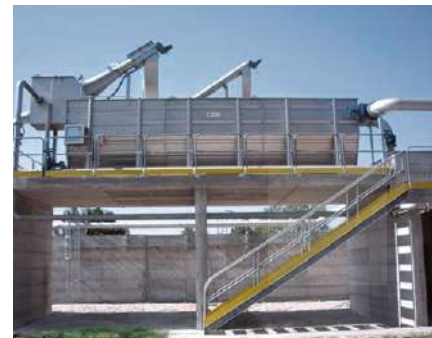
Municipal wastewater treatment plant
