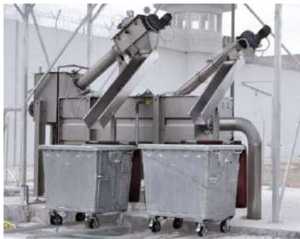
Prison wastewater treatment
