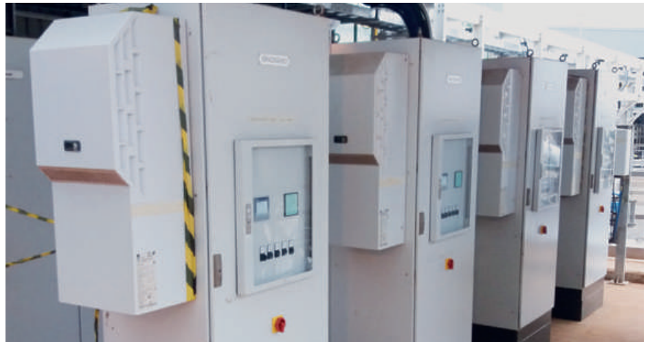
Fig. 4: Geiger® ICCP Corrosion protection cabinets at a power plant in Ghana
