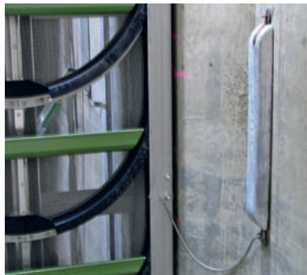
Fig. 6: Protection of a Geiger MultiDisc® Screen by means of sacrificial anodes
