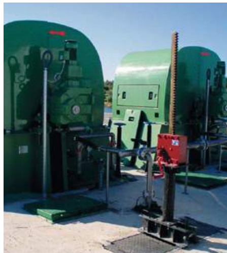
Travelling Band Screen Dual Flow Pattern
