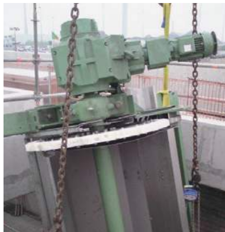
Installation of a Geiger® Travelling Band Screen Driving Shaft
