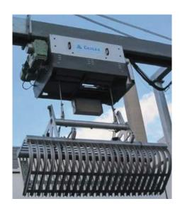
The Geiger® Claw Screen with travelling unit and claw bucket operates on a monorail track between the bar racks and the dumpster position. Mild steel supporting structures, including curved track sections can be tailored to fit into the claw bucket's immediate surroundings.
