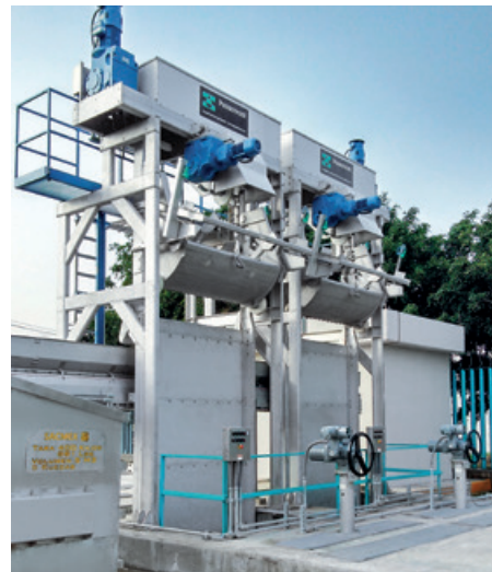
Passavant® Cable-Operated Bar Screens COB-XXL with Passavant® Penstocks (2000 x 2000 mm)
