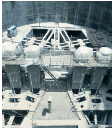
Passavant® Cable-Operated Bar Screens COB-C Passavant® Penstocks (1200 x 3500 mm)
