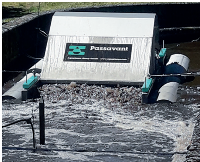
Passavant® Surface Brush Aerator Mammutrotor® Lago for oxidation ponds
