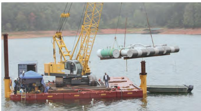
Installation eines Johnson Offshore Intake Systems™ (JOIS™)
