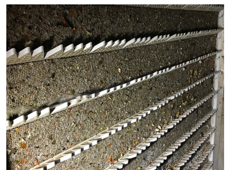
Blinding of filter elements
