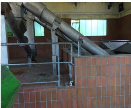
Existing plant / Condition before the renovation
