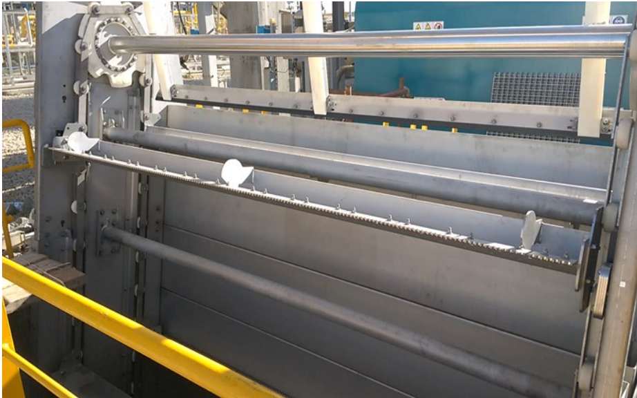
Geiger® Revolving Chain Screen during commissioning phase
