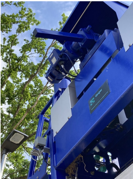
Geiger® Cable Operated Bar Screen (above deck level)
