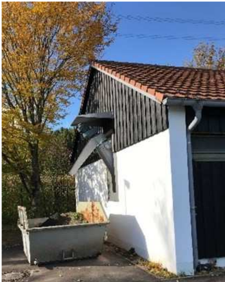
Exterior view of the screen building (Sand discharge conveyor with wall penetration)
