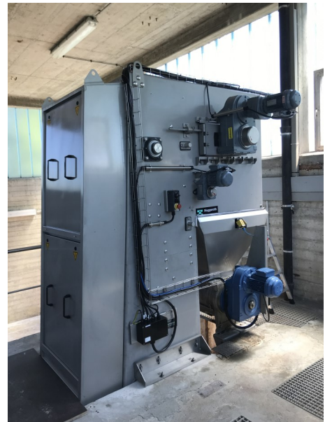
Closed front doors during operation
