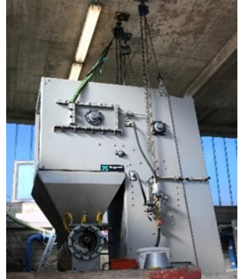
Side view of the screen (Flange of the screenings discharge)
