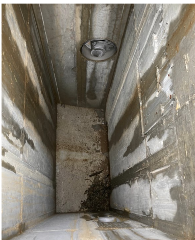
Discharge screenings chamber
