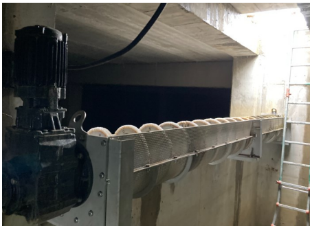
Noggerath® overflow screen OVF at the combined sewer overflow
